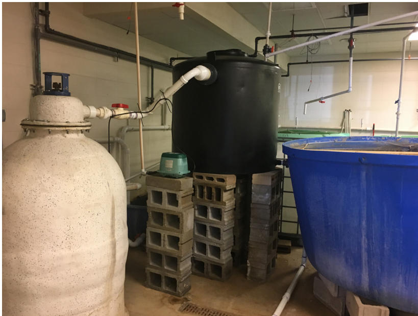
Figure 10. Installation of new biofilters built with donated materials in 2018.
