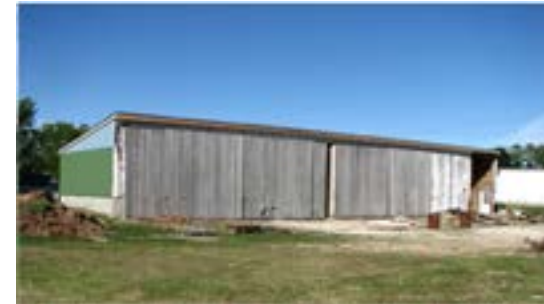
Figs. 8 and 9. A dilapidated agricultural storage building with pitched roof that would become the future model 3. (P. Wilborn, 2011.)
