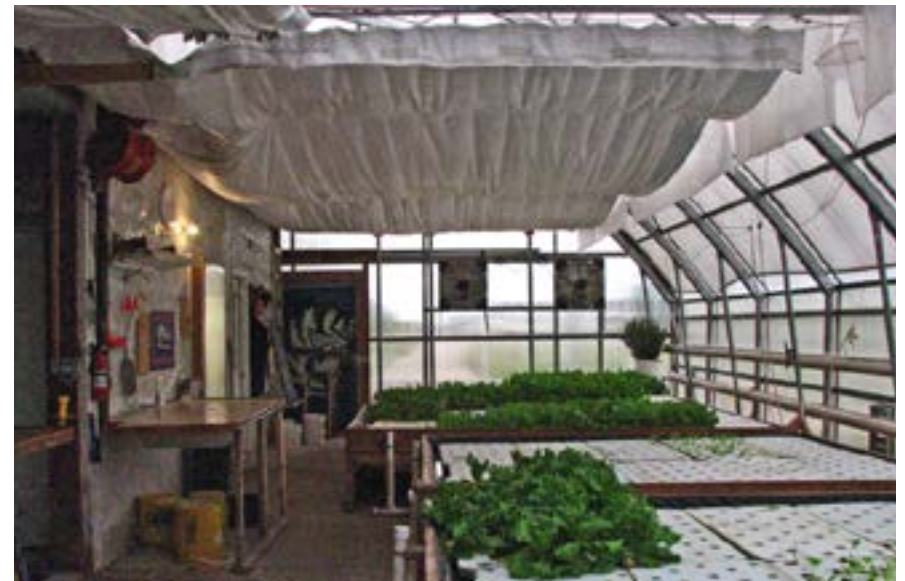
Figs. 12 and 13. Installation and functionality of retractable thermal curtains. (P. Wilborn, 2012.)
