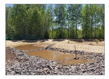
The first pond is designed to be a wetland at all times — it receives all the runoff and most of the sediment. The second pond acts like a wetland when lake levels are high, but will act more like a bio-infiltration basin during low-water years. For most small, frequent rains there may be little or no flow out of the second pond. Over time, two distinct plant communities should develop in each of the ponds because of the differences in hydrology.
