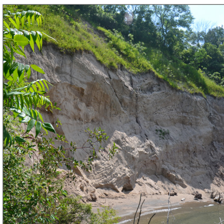
Severe Toe Erosion
