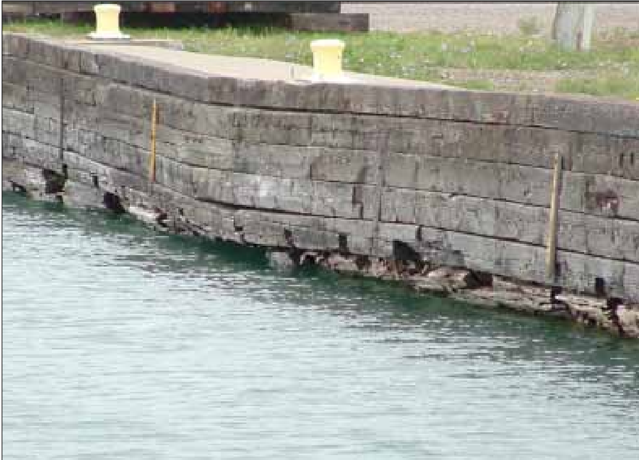
Figure 3: Timber Bulkhead Wall Failure on Lake Superior.
