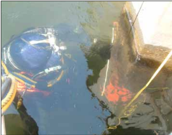
Figure 4: Typical Diver Inspection of Steel Bulkhead Wall.
