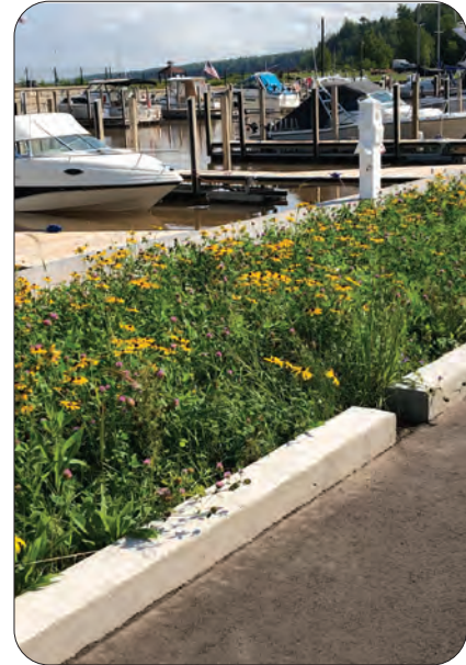
Bioretention basins with native plantings at Saxon Harbor Marina. Photo credit: Theresa Qualls, Wisconsin Sea Grant.
