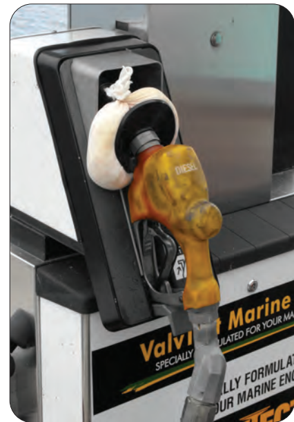
Absorbent pad on fuel pump at Pikes Bay Marina. Photo credit: Gene Clark, Wisconsin Sea Grant.
