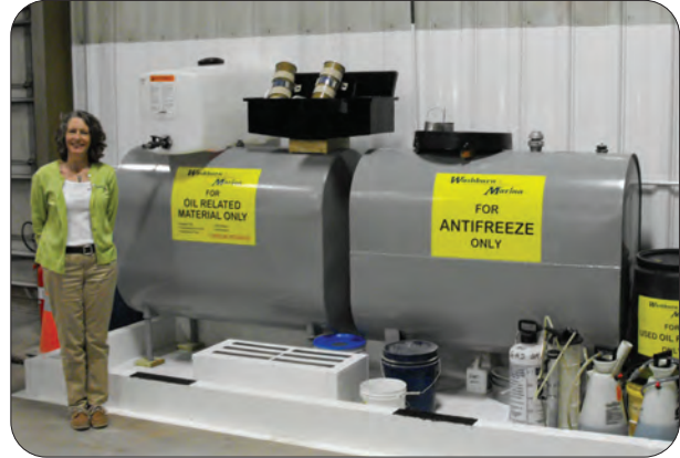
Waste containers and containment at Washburn Marina. Photo credit: Gene Clark, Wisconsin Sea Grant.
