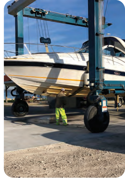
Pressure-washing boats on wash pad with catch basin that discharges to wastewater treatment facility. South Bay Marina. Photo credit: Theresa Qualls, Wisconsin Sea Grant.
