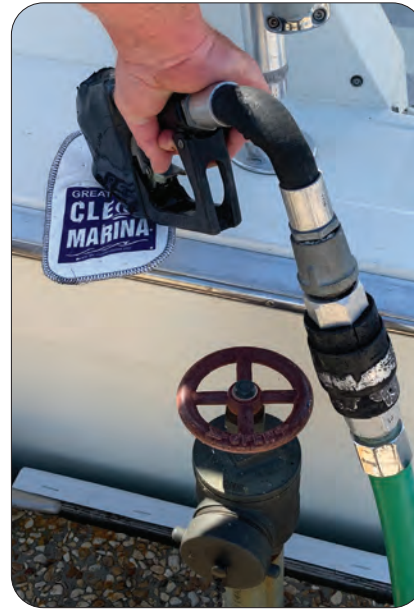
Absorbent fuel bib at Port Washington Marina. Photo credit: Mari Mitchell, Wisconsin Sea Grant.
