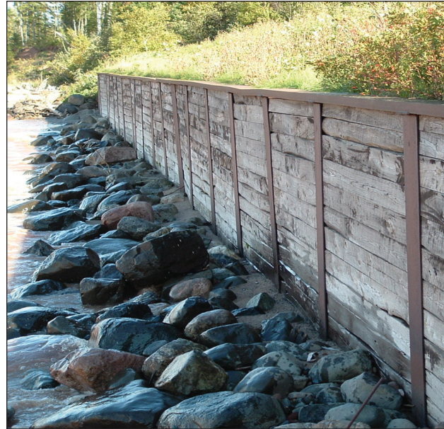
Figure 3: Timber soldier pile wall (Gene Clark/UW Sea Grant Institute).
