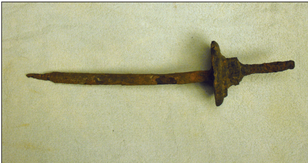
Figure 9: Corroded timber crib connection steel pin (Gene Clark/UW Sea Grant Institute).
