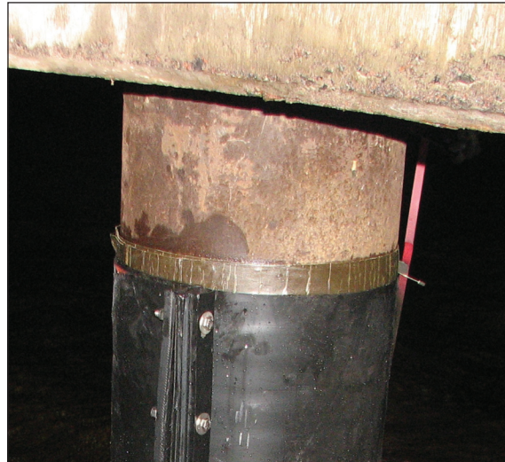
Figure 15: High-density polyethylene jacket option shown on steel pile (Gene Clark/UW Sea Grant Institute)
