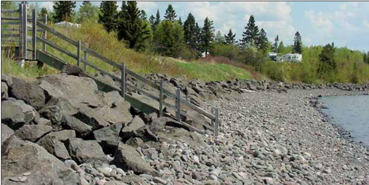
Figure 1: An example of a Great Lakes revetment
