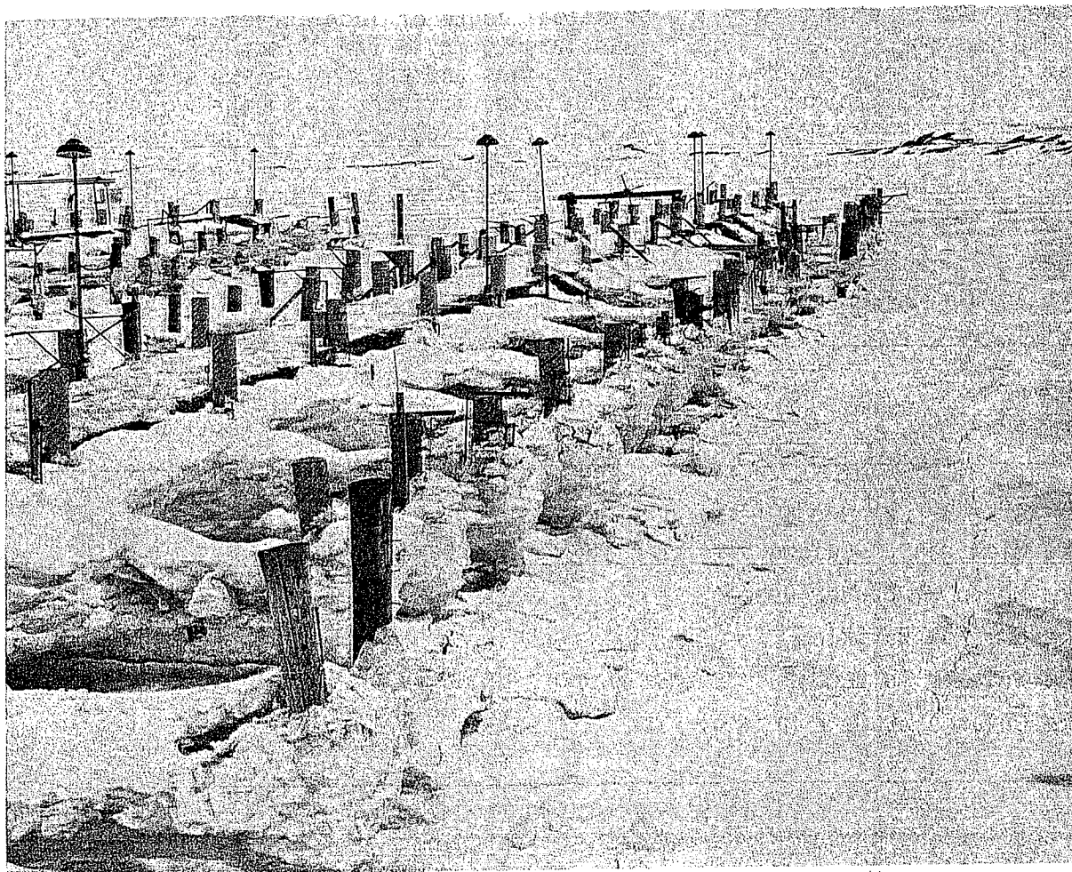
FIGURE 6.3: Lake Erie Marina Covered with Ice Left by Receding Water Setup.
