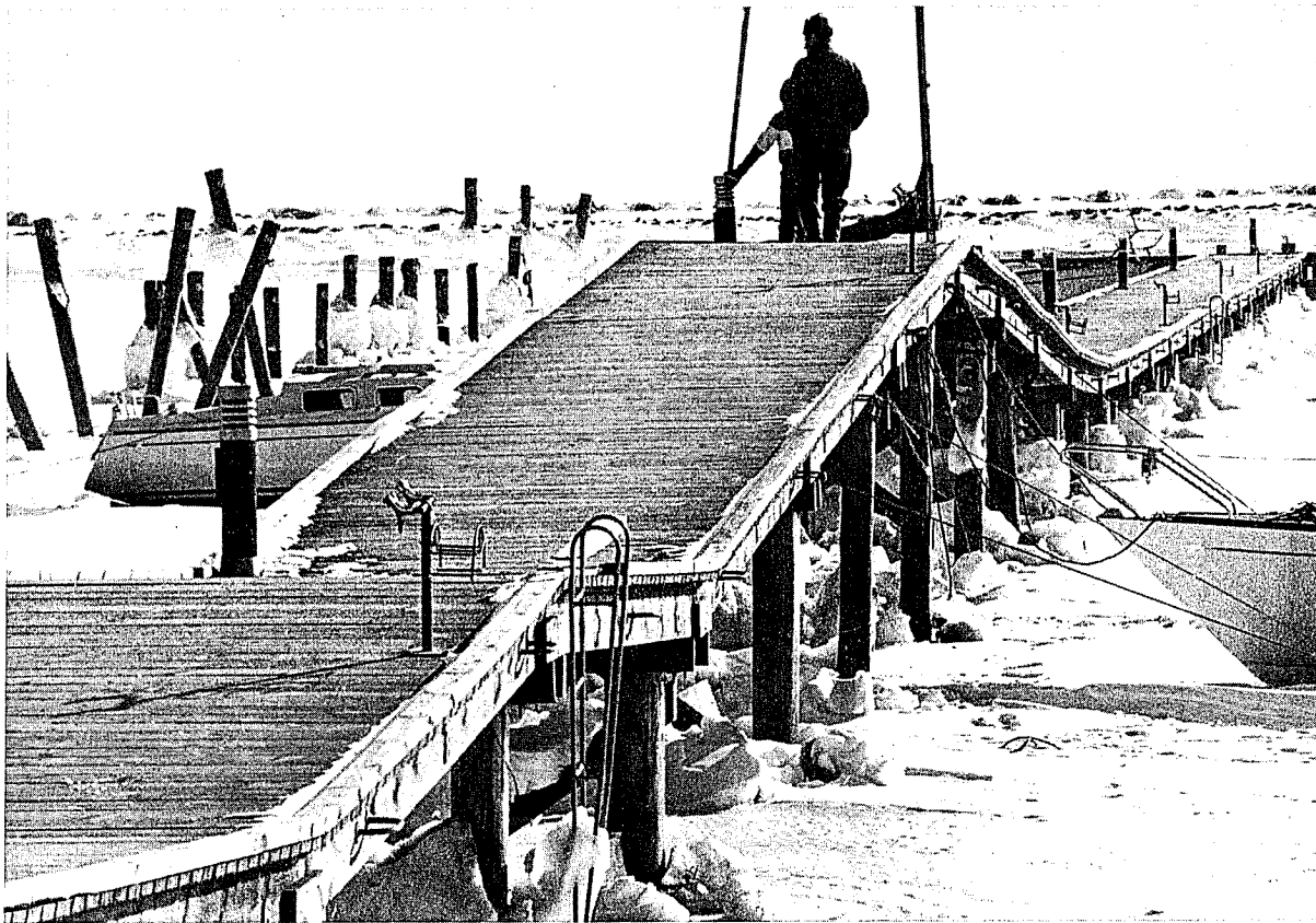
FIGURE 13.2: Timber Head Pier Damaged by Ice
