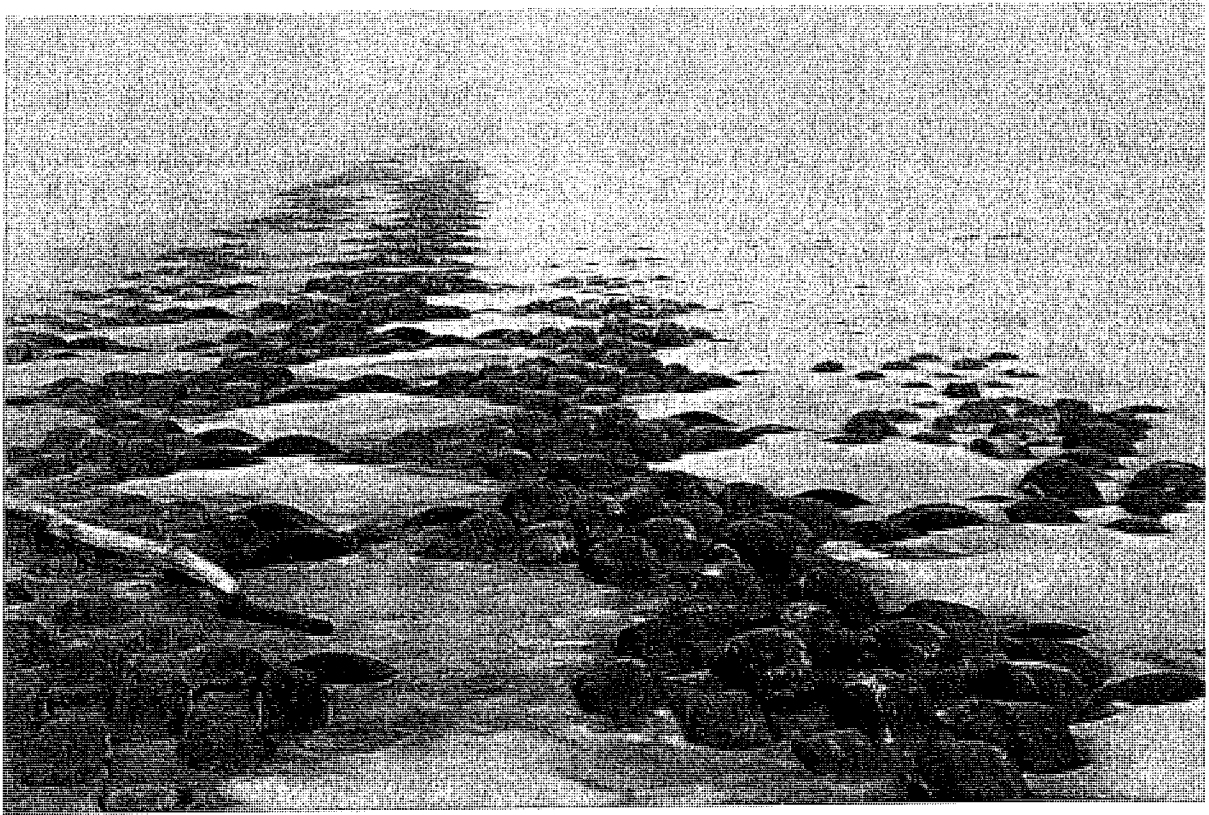
FIGURE 9.9: Floating Tire Breakwater (FTB) Wintering in Ice
