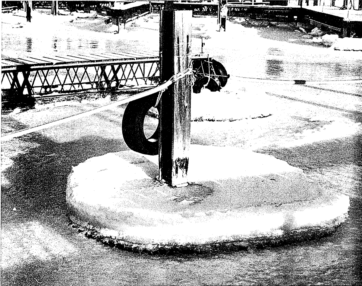
FIGURE 11.2: Large Ice Collar on Steel Harbor Piling
