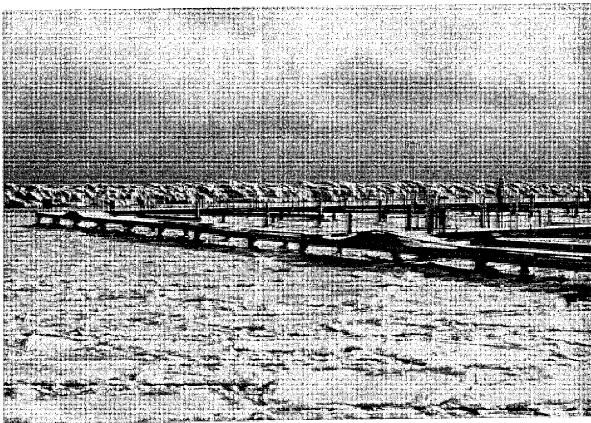
FIGURE 3.5: Broken Ice Cover Moving through Marina Dockage
