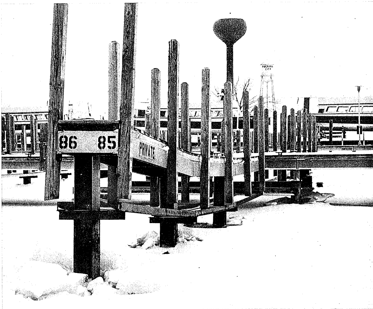
FIGURE 11.1: Steel Harbor Piles Uplifted by Ice
