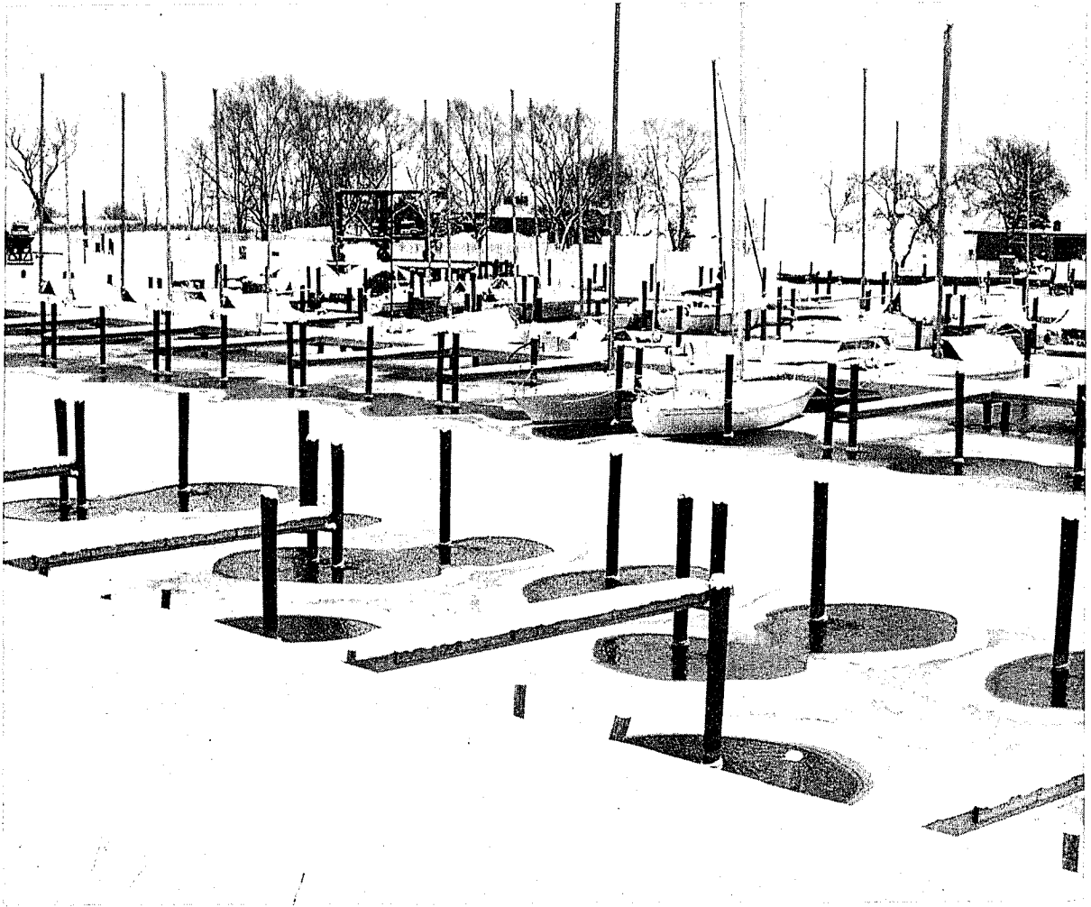
FIGURE 8.2: Compressed Air Ice Suppression System
