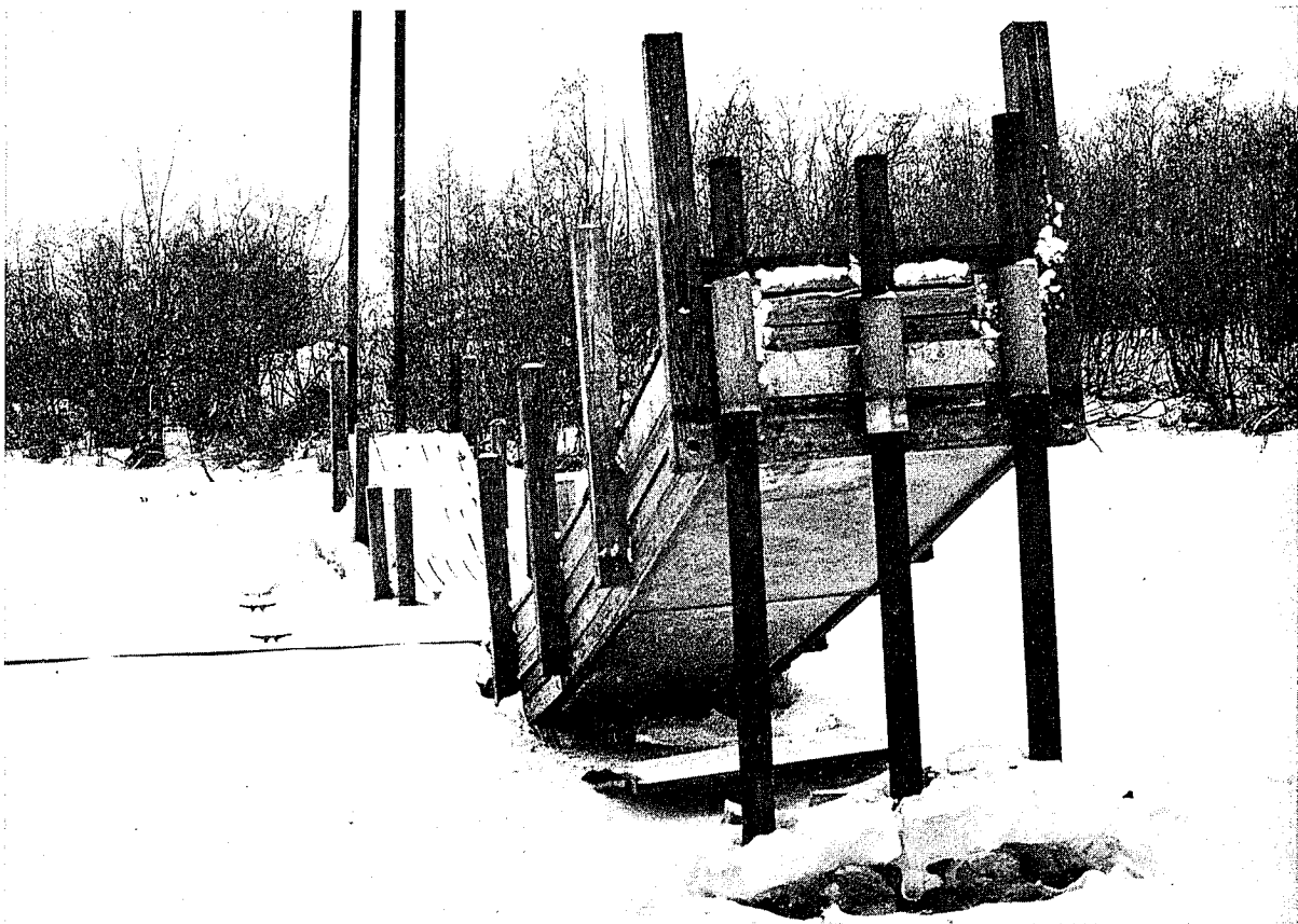
FIGURE 9.6: Floating Dock Damaged by Lifting Spuds
