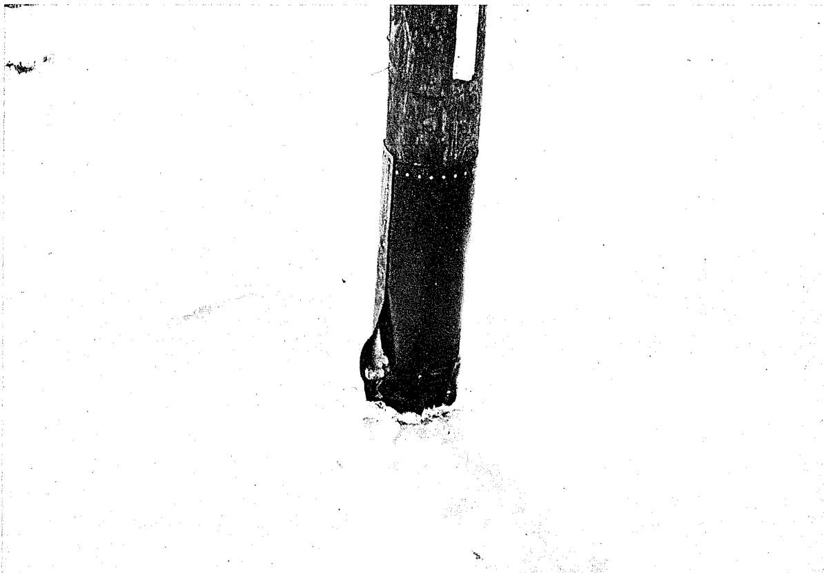
FIGURE 11.4: Black Polyethylene Pile Wrapper
