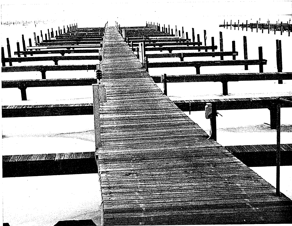
FIGURE 3.6: Small-Craft Harbor Head Pier Bowed by Thermal Ice Pressure
