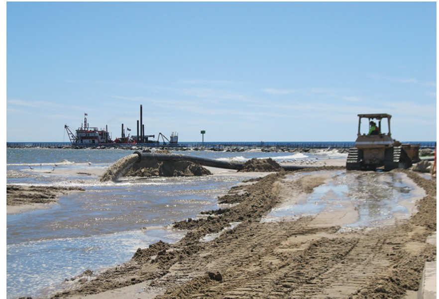
Clean, coarse-grained sediment dredged from the Two Rivers Harbor in Wisconsin is pumped to the placement site and spread across the beach with heavy machinery. Jim Killian
