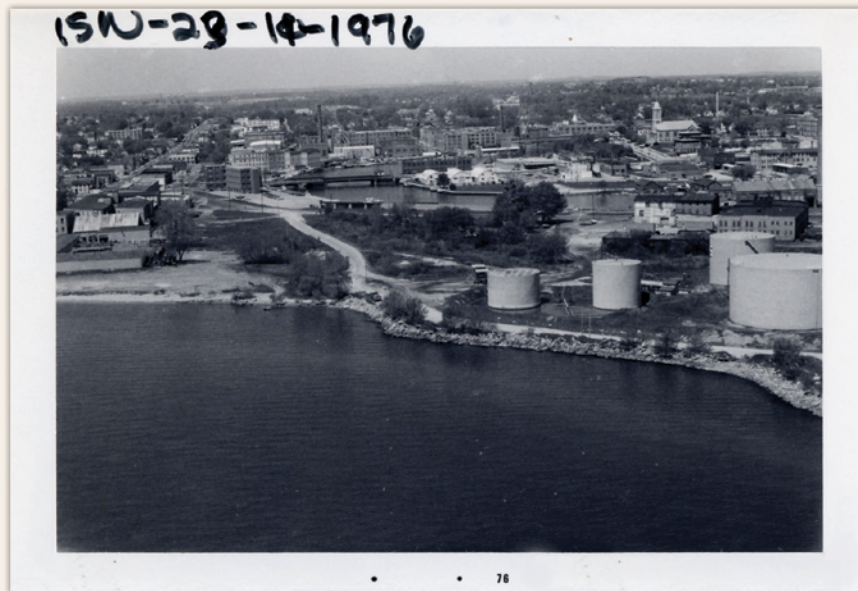
Before Nourishment (1976) Concrete rubble on the shoreline provided erosion protection for oil storage tanks. Dave Mickelson
