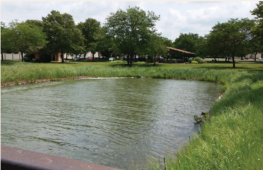
After Edging helped native vegetation establish to stabilize the shoreline. Visual appeal has also improved. Erie Soil and Water Conservation District
