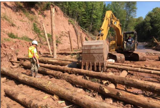
Earthwork in 2021 on Fish Creek
