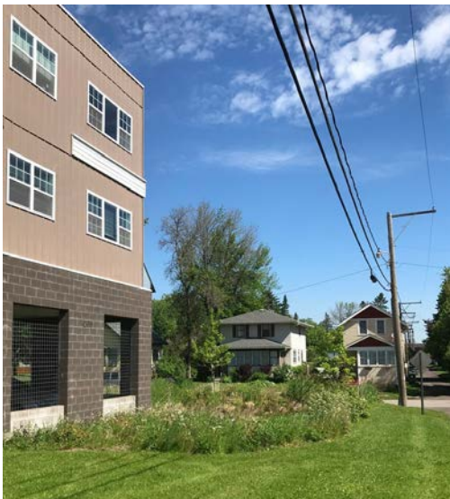
Green infrastructure for stormwater management at new multi-family complex, city of Superior
