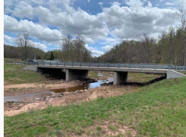
Wider stream passage at reconstructed bridge providing resilience against future strong storms, Saxon Harbor
