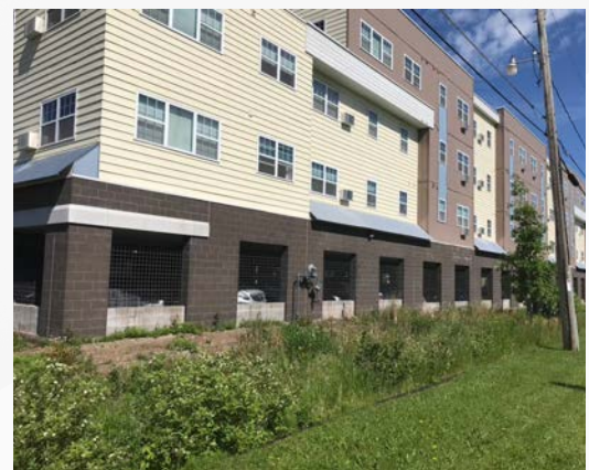
Bioretention, city of Superior
