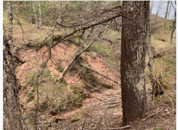
Stream erosion in a tributary to Lake Superior, Saxon Harbor
