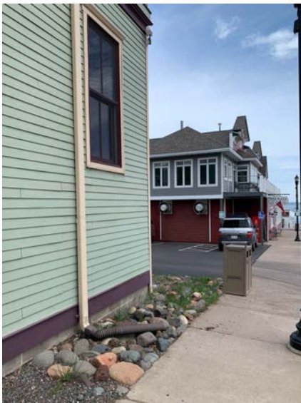
Downspout redirection, city of Bayfield
