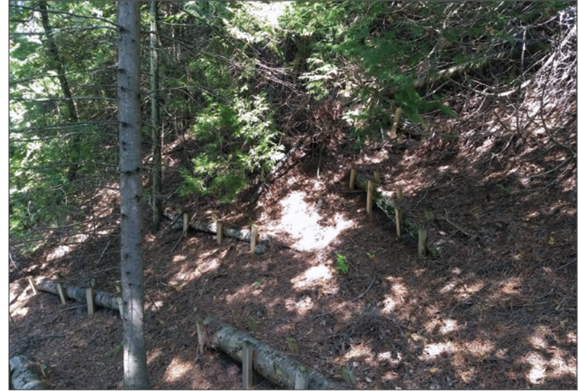
Brush and logs staked in to the bluff to slow the flow of surface water runoff. Adam Bechle
