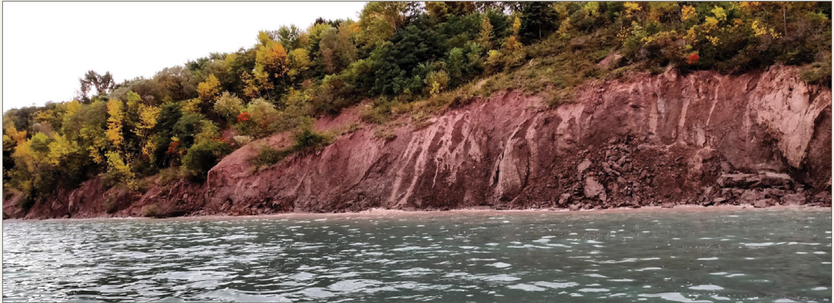
Severe toe erosion. Chin Wu
