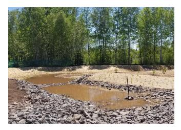
The first pond is designed to be a wetland at all times — it receives all the runoff and most of the sediment. The second pond acts like a wetland when lake levels are high, but will act more like a bio-infiltration basin during low-water years. For most small, frequent rains there may be little or no flow out of the second pond. Over time, two distinct plant communities should develop in each of the ponds because of the differences in hydrology.
