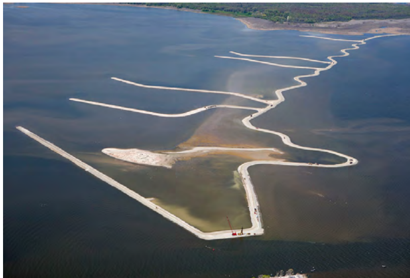
Figure 91: Cat Island spine construction, May 2013.
